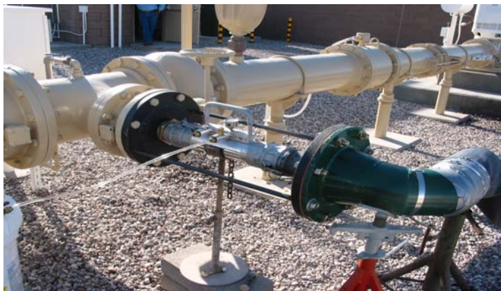
VENTURI EDUCTOR SYSTEM TO FEED ASCORBIC ACID
