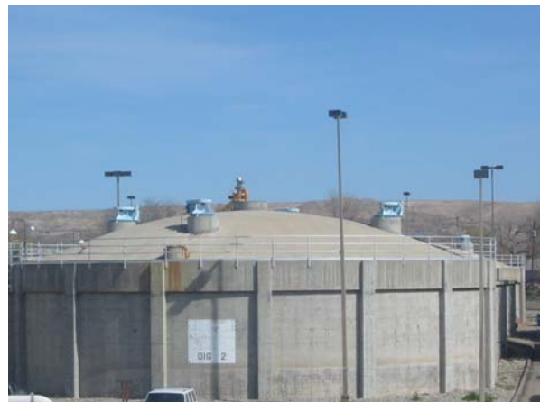
Primary digester with mechanical mixers
